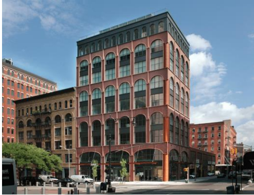
408 Greenwich Street uses unadorned terracotta arches as a modern interpretation of the traditional masonry buildings found throughout its Tribeca neighborhood. Image: Jimi Billingsley.
